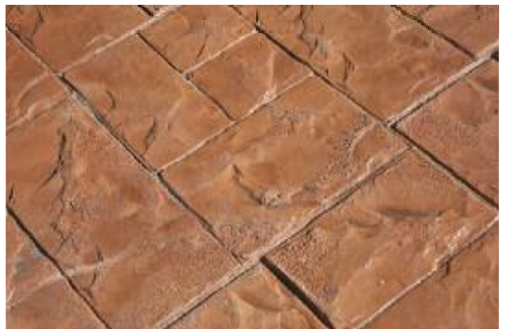
Detail of "Roman Opus" embossed concrete
