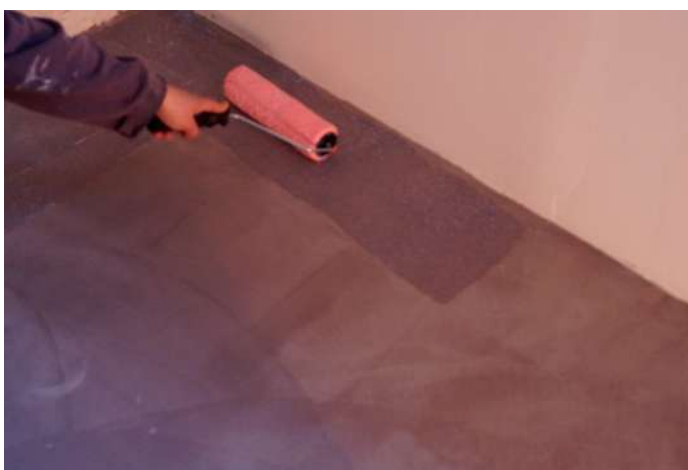
After dusting the surface, apply the pores mouth. On a large surface, use a 500 mm roll or a microfiber mop. Let dry from 2 to 4 hours.
