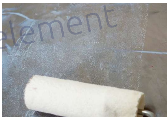
Smooth with the special varnish roller in order to standardize the application.
