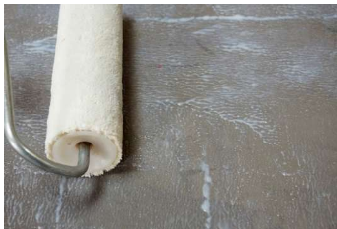
Let dry for at least 6 hours and apply the 2nd coat.
