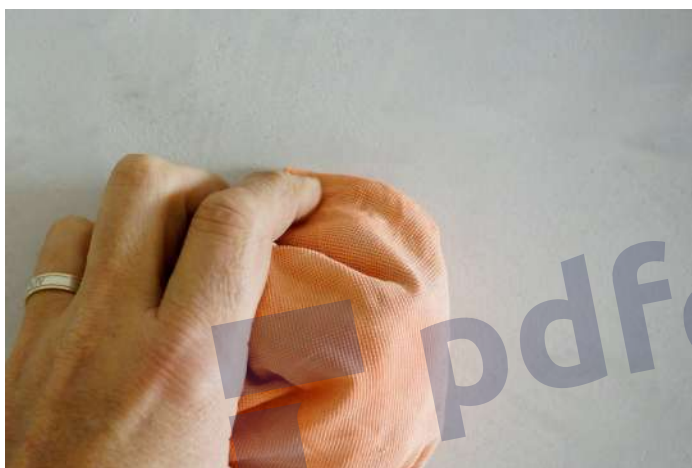
Wipe the excess wax with a soft cloth in order to remove any traces of application of the wax.
