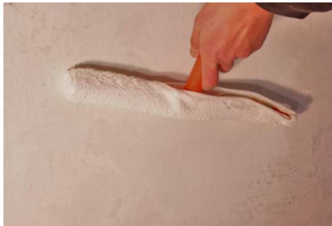
Apply the wax with a cloth or a wet broom Work from the bottom to the top
