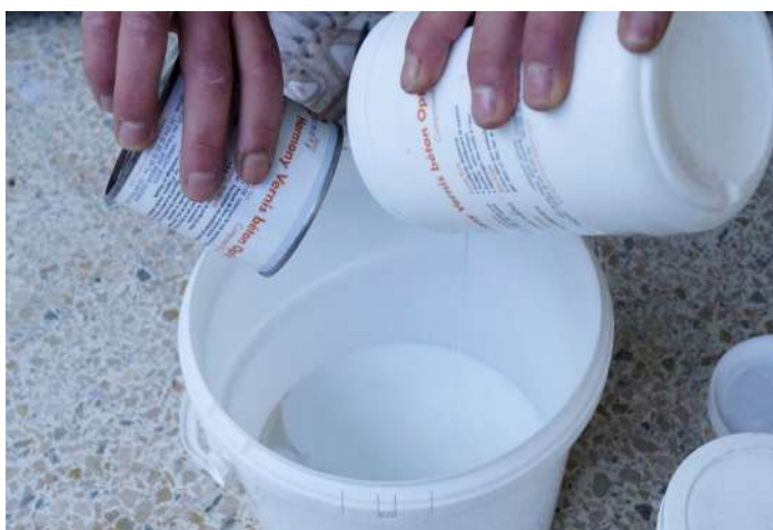
Pour the 2 components of the Optimum varnish after having weighted them in a clean bucket.
