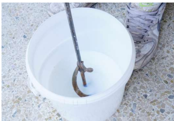
Mix the 2 components with slow speed for 1 min. Life time of the mixture +/- 45 mns depending on the ambient temperature.
